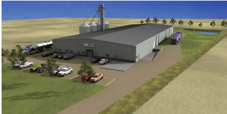
Saskatoon Plant Under Construction (Start-up January 2009)
